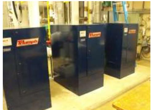
These boilers are controlled by an integrated Honeywell Microprocessor-Based Control System that provides PID Temperature Control and Flame Management.
