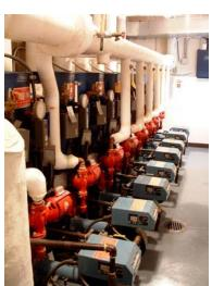
Al Grode of G & R Controls, in Sioux Falls, SD, has been involved with this facility since 1995 and continues to provide service for the facility under an annual contract. The solution to the leaking boiler was simple. As the original sixteen boilers were still in place, but with their original atmospheric burners, it was decided to replace all of them with NEW TRIAD GPS-300-SH-HEP & GPS-300-SH-C-DWH-HEP boilers with more efficient Powerflame power burners.
