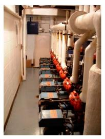
had a TRIAD Series 8900 lead-lag sequence panel installed to control the sequencing of the boilers based on outdoor and return-water temperatures.
