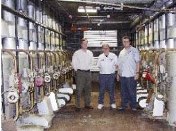
small size, these vessels have 12 gauge firetubes rolled into 3/8" thick tube sheets, with a wall thickness of 1/4". Any boiler replacement will be as simple as it was 40 years ago – by the use of a hand truck, into the elevator, up to the penthouse, and through the 30" doorways.
