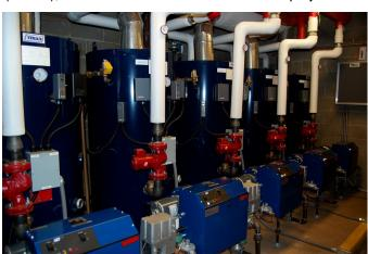
Hildreth of THCO suggested the installation of 10 new Triad Boilers, consisting of five Series 300-SH boilers firing at 399MBH and five Series 900-SH boilers firing at 900MBH. Replacing the old boilers was a good opportunity for Grinnell to get rid of the hassles of firing with oil, and instead switch to cleaner burning natural gas. The Series 300¢s were fired by Powerflame X4-400 burners and the Series 900¢s were fired by Powerflame JR30 burners.
